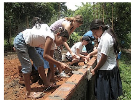
Nicaraguan community members working with foreign volunteers to construct school wall
